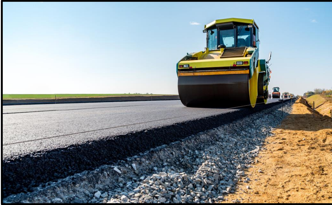
Example of roadway paving
